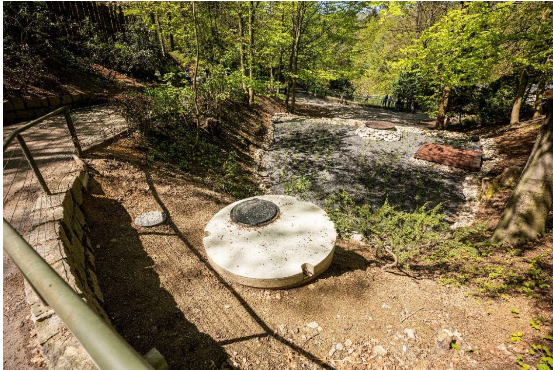
Finished constructed wetland with pulse and pumping shaft.
